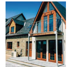
Tower Ridge Courtyard in Schottland (GB)
